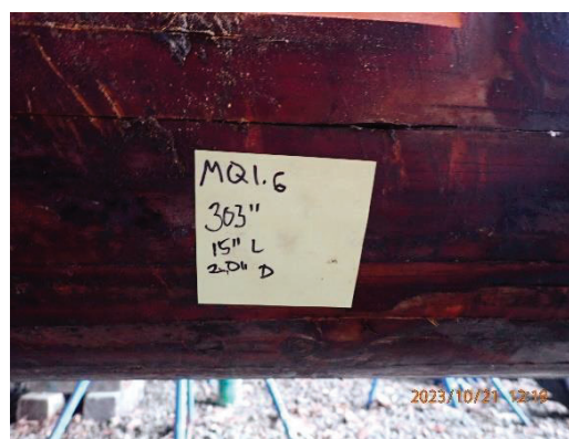
Figure 32 – Check Number 1.6 (15" length x 2" depth). Probing revealed soft wood.
