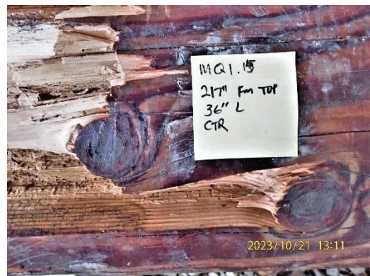
Figure 60 – Check Number 1.15 (36" length). Probing revealed soft wood, penetrating into the center without resistance.
