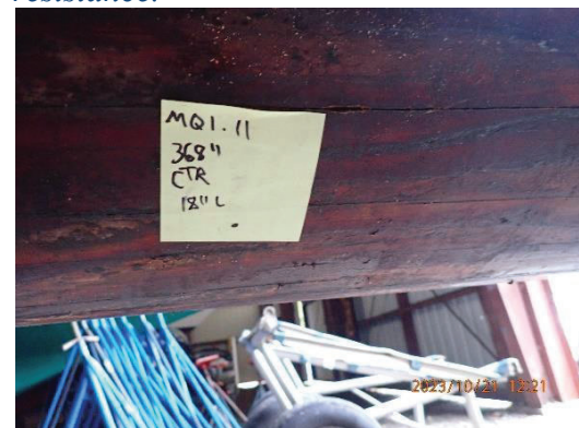
Figure 46 – Check Number 1.11 (18" length). Probing revealed soft wood, penetrating into the center without resistance.
