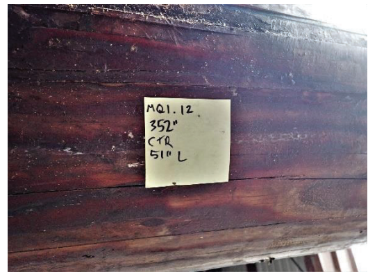
Figure 44 – Check Number 1.12 (51" length). Probing revealed soft wood, penetrating into the center without resistance.
