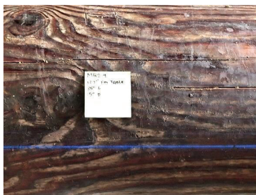
Figure 13 – Check Number 2.9(35" length x 1/2" depth). Probing did not reveal soft wood
