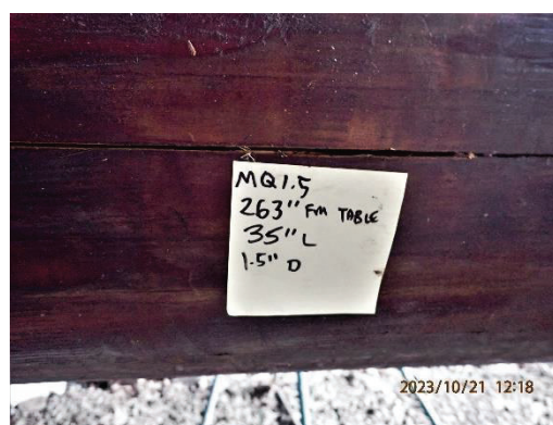
Figure 34 – Check Number 1.5 (35" length x 1 ½" depth). Probing revealed soft wood.
