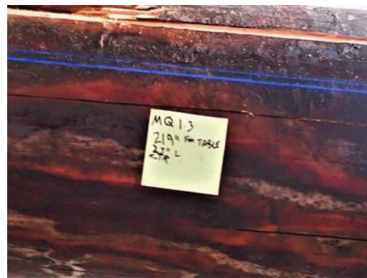
Figure 21 – Check Number 1.3 (23" length). Soft wood apparent with probing. Probe was able to penetrate into center without resistance.
