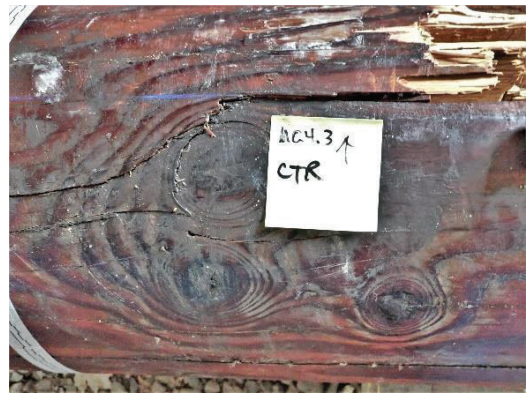
Figure 52 – Check Number 4.3 (57" length) Probing revealed soft wood, penetrating into the center without resistance.
