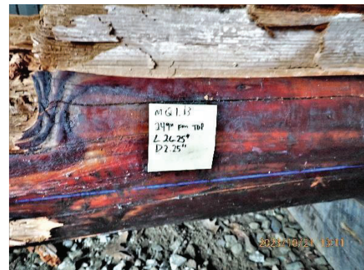
Figure 54 – Check Number 1.13 (26" length x 2 1/4" depth). Probing did not reveal soft wood.
