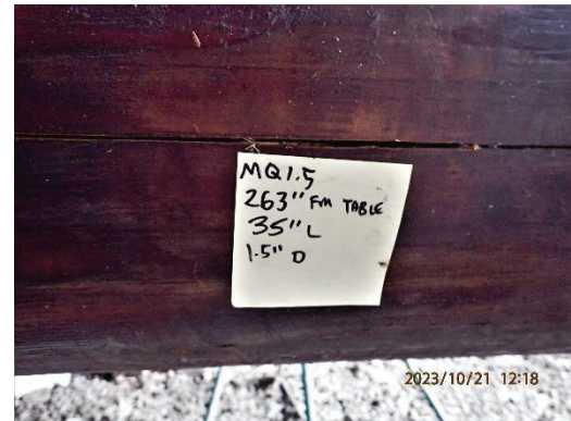
Figure 29 – Check Number 1.5 (35" length x 1 ½" depth). Probing did not reveal soft wood.
